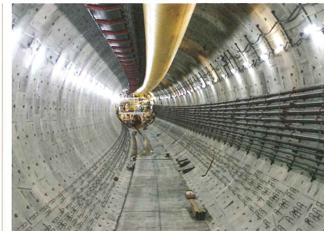
Photo of tunnel posted after the maintenance stop
