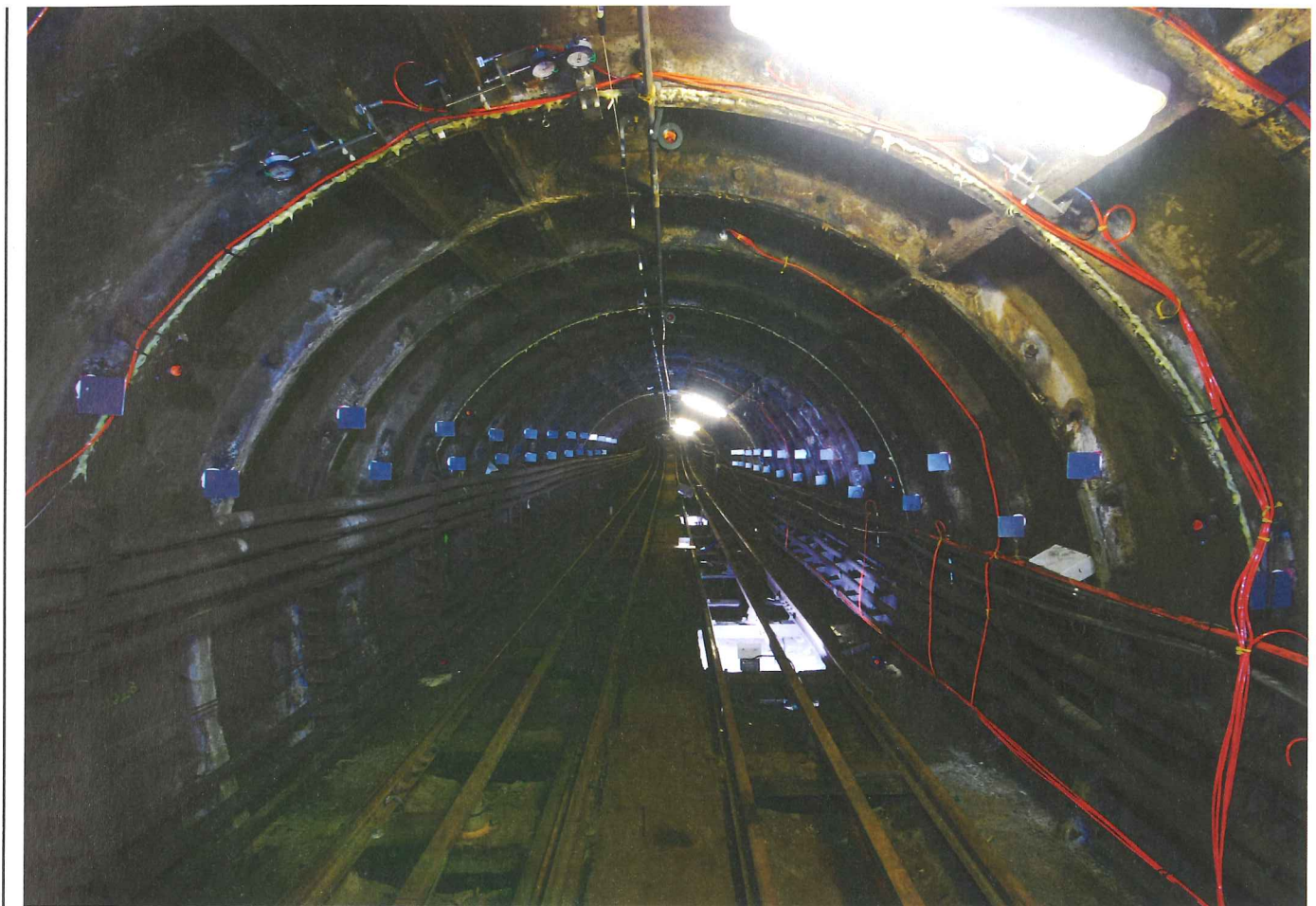
Above: The Royal Mail Tunnel
