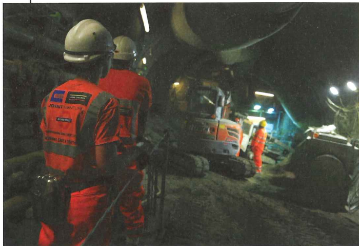
Top: Engineers carrying out checks prior to the construction of a secondary lining invert slab in a tunnel
