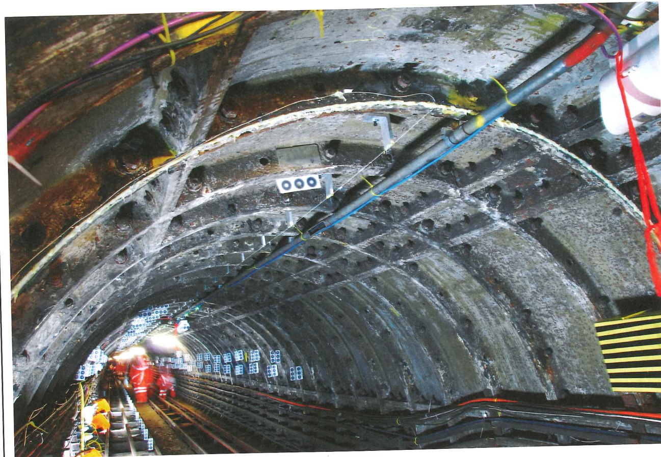
Above: The Royal Mail Tunnel
