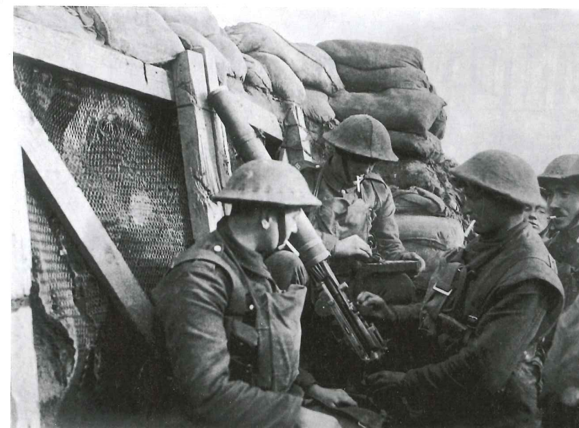
Below: A machine gun emplacement on a front line trench
