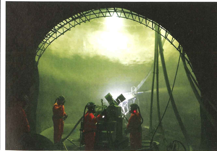
Below: Secondary lining spraying underway in Shaft 3, the final section of sprayed concrete lining on BSSU
