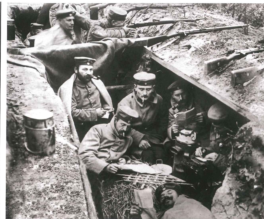
Above: Positioned below the lip of the trench, soldiers are protected from blast shockwaves and shrapnel
