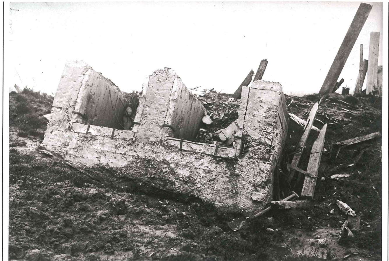
Above: Concrete fortification destroyed by a tunnelled explosives cache. Such structures could be several metres underground
