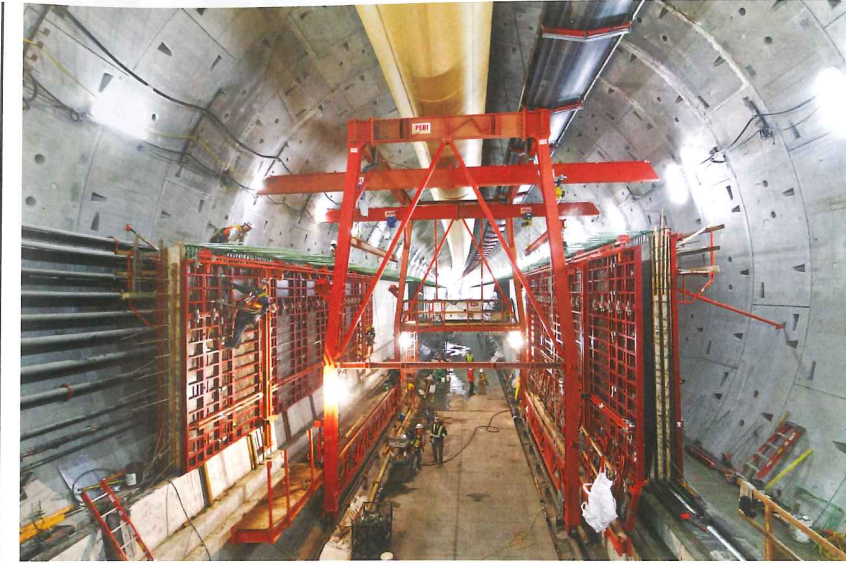
Above: Deck casting formwork in bored tunnel PHOTO: WSDOT
