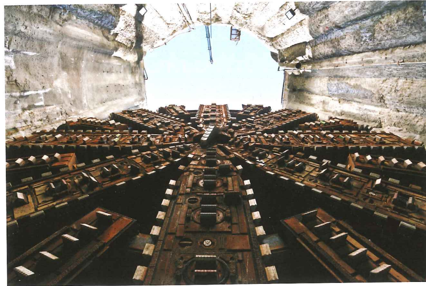
Above: The TBM in the access shaft PHOTO: WSDOT
