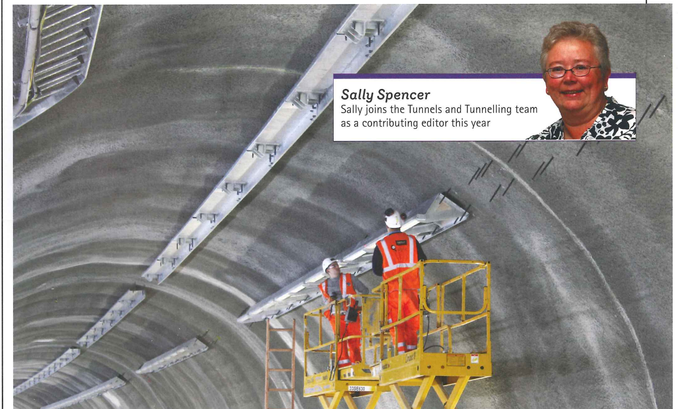
Below: Platform Edge Screen brackets are securely held in position by Excalibur M20 studbolts
