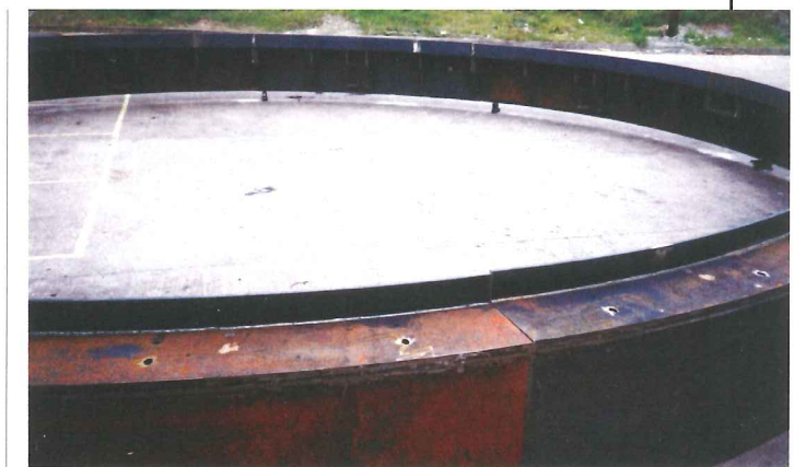
Top: Underpinning showing trimming.
