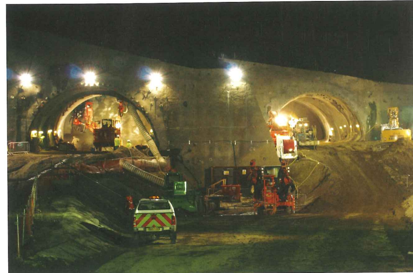
Above: The Hindhead Tunnel project
