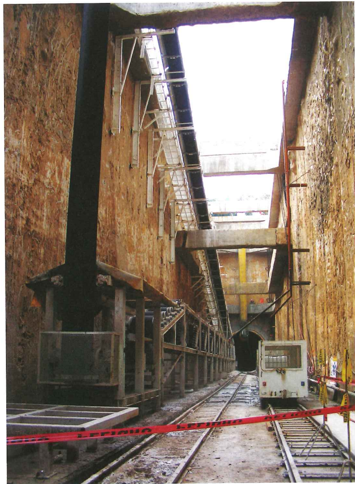
Above: The launch shaft and continuous conveyors
