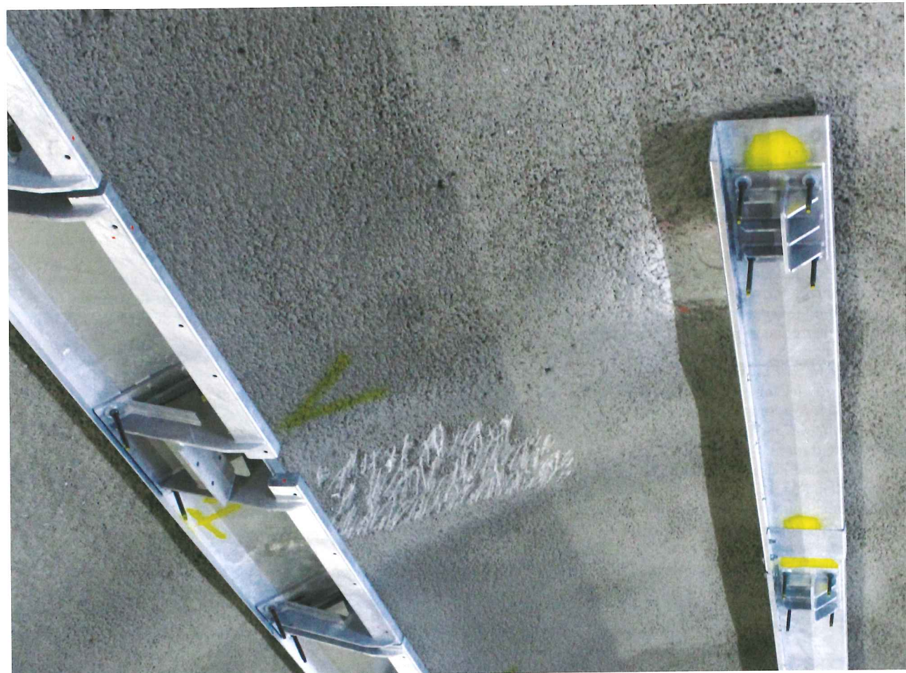
Above: Platform edge screen brackets after adjustment for line and level
