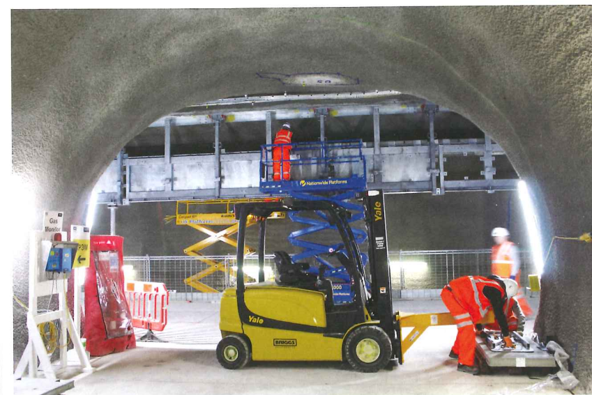
Below: Steelwork in position; GFRC panels can be placed
