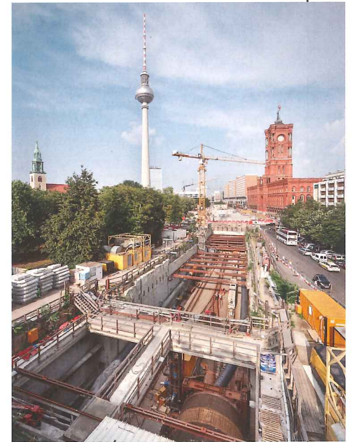
Ongoing work for the Berlin U5
