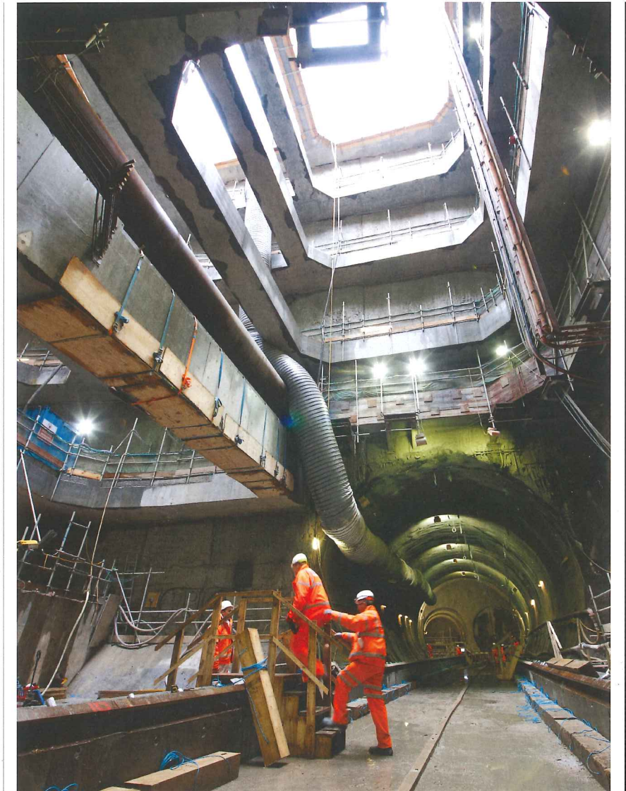
Above: Main tunnel excavation has completed on London's Crossrail project
