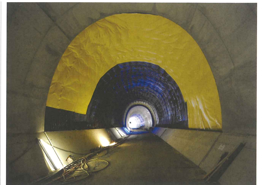
Above: Sealing work ongoing in October 2012
