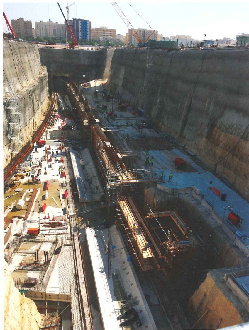
Above: Construction work in Doha
