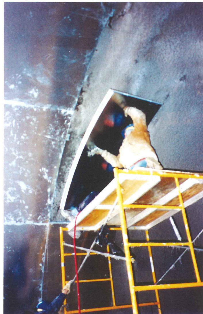
Above: Figure 5. Installation of premanufactured panels
