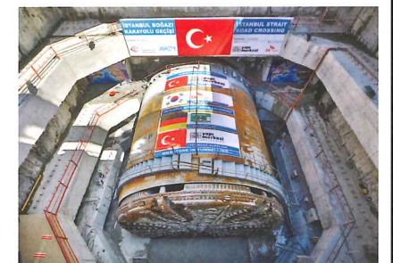
The TBM was named Yıldırım ('Lightning') after an Ottoman Sultan
