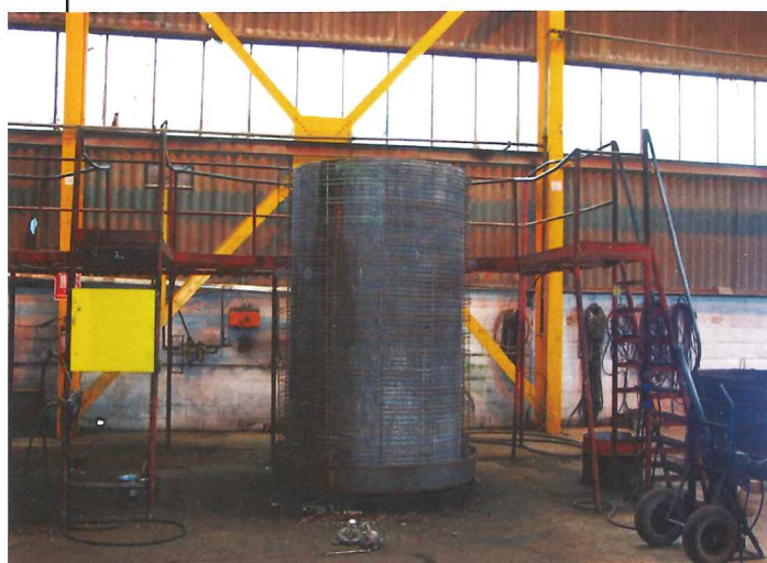
Below: Cage reinforcement in a pipe jacking pipe
