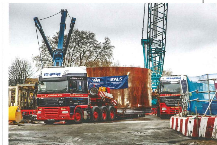
Above: Heavy loads handling for European tunnelling projects
