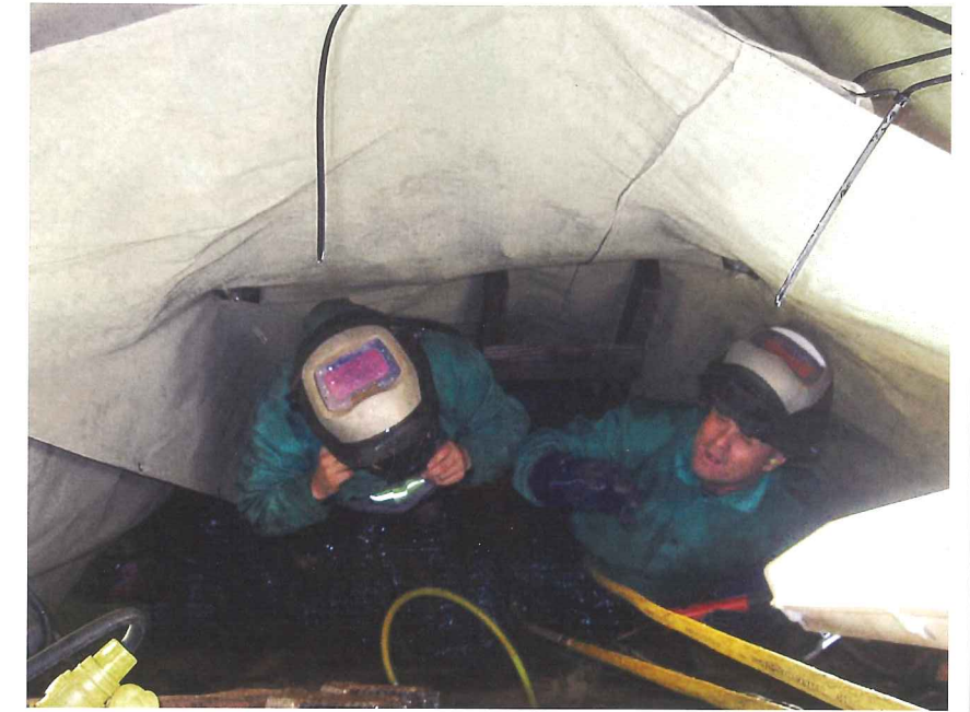
Above: Crew members out front of the TBM
