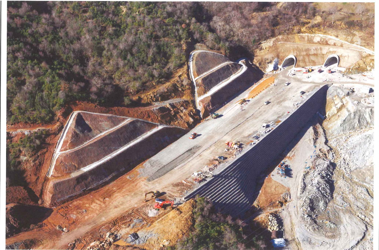
Above: The Albania Krrabe Tunnel on the Elbaban Motorway
