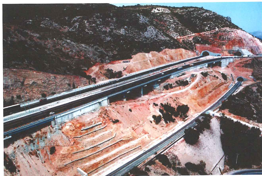
Below: The Kakia Skala Tunnels on the Pathe Motorway
