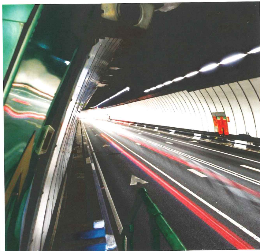
Below: The Kingsway Tunnel is due to undergo upgrade works
