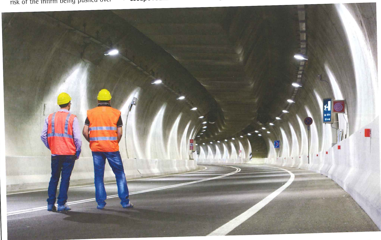
Below: Image illustrating an easily accessible escape route
