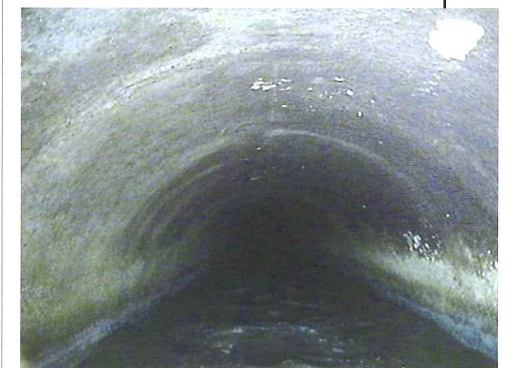
Right: Figure 3, a screenshot from the CCTV monitoring of the YDSS during jet grouting operations
