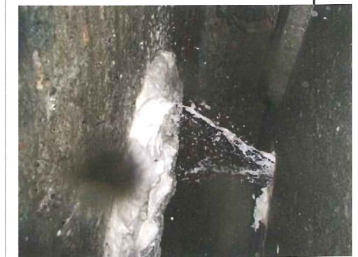
Right: Figure 4, testing GCS lines after repair in the headwall
