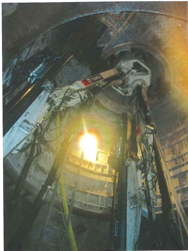
Below, right: Mucking portion of the shaft excavation cycle
