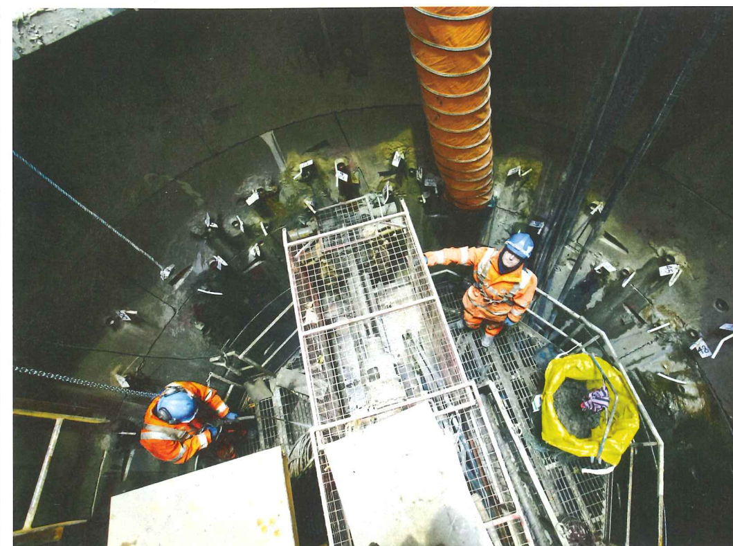
Left: Work on Bond Street Station in London, UK. See page 36
