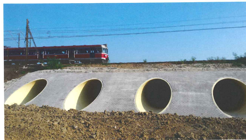
Above: The culvert is now in operation
