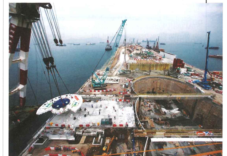
Below (bottom): TBM launching shaft is prepared
