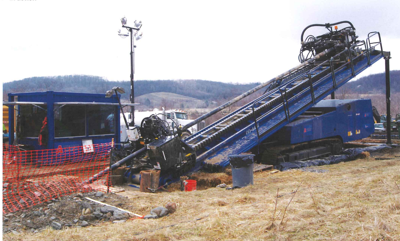
An American Augers HDD rig in action
