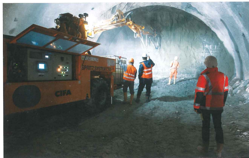
Above: Excavation face on the Brenner Base Tunnel project
