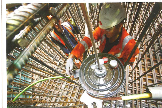
Work underway at the Fisher Street Crossrail site
