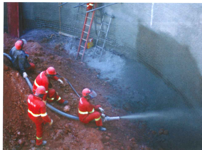
Above: Figure 4, Application of sprayed concrete. Both photos depict Access Jardins in October 2012
