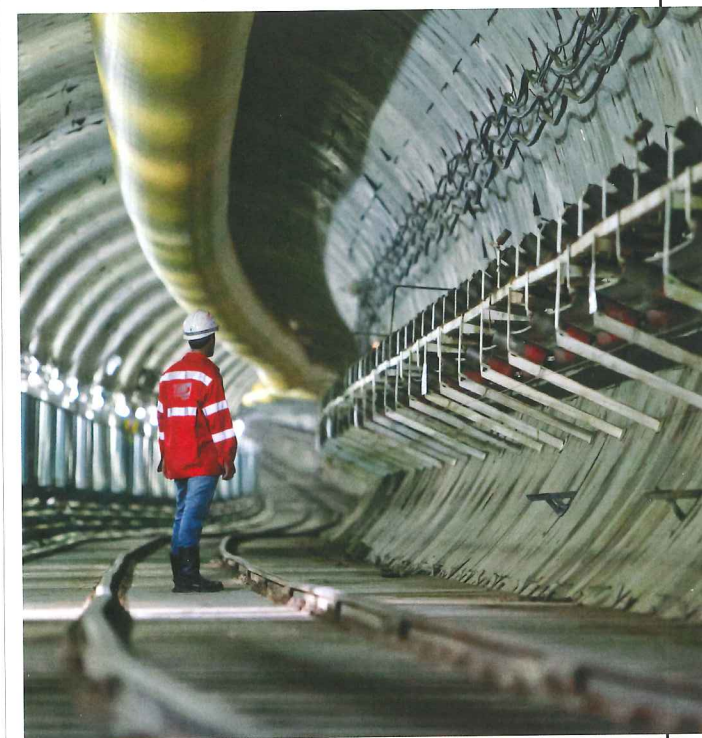
Above: One of the longest continuous conveyors ever provided by Robbins, for the AMR project in India. Two sets of conveyors will extend up to 22km each in several flights
