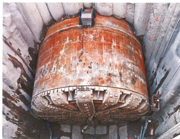
Excavation was halted over a year ago
