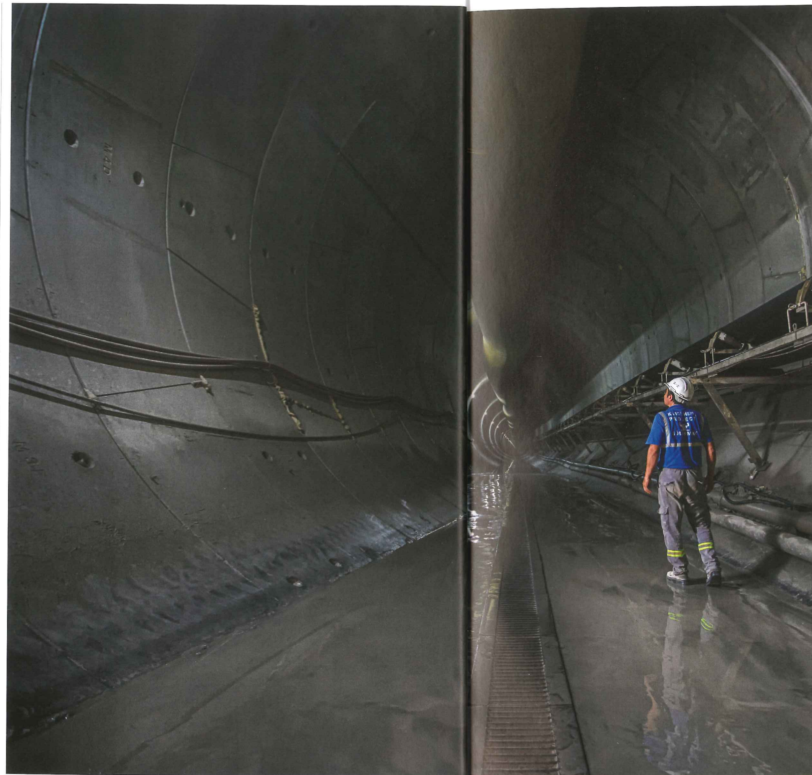
Above: At Turkey's Kargi HEPP, a worker pauses while a side-mounted conveyor works to remove mixed ground
