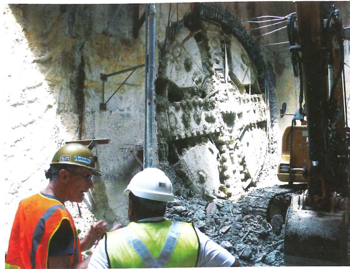
Both: TBM assembly and operations in confined space
