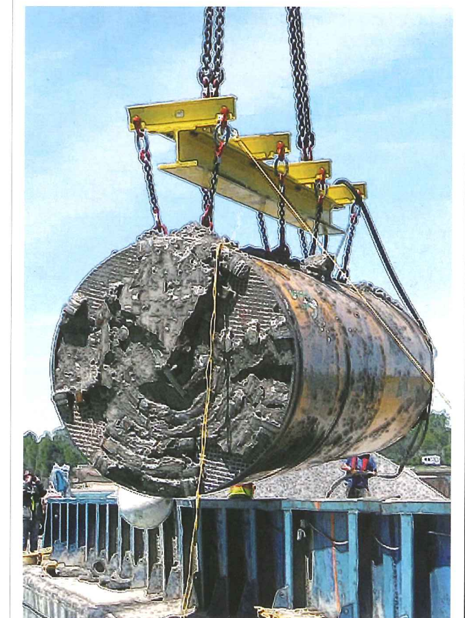
Below: Crews remove the TBM from Lake Huron off a barge
