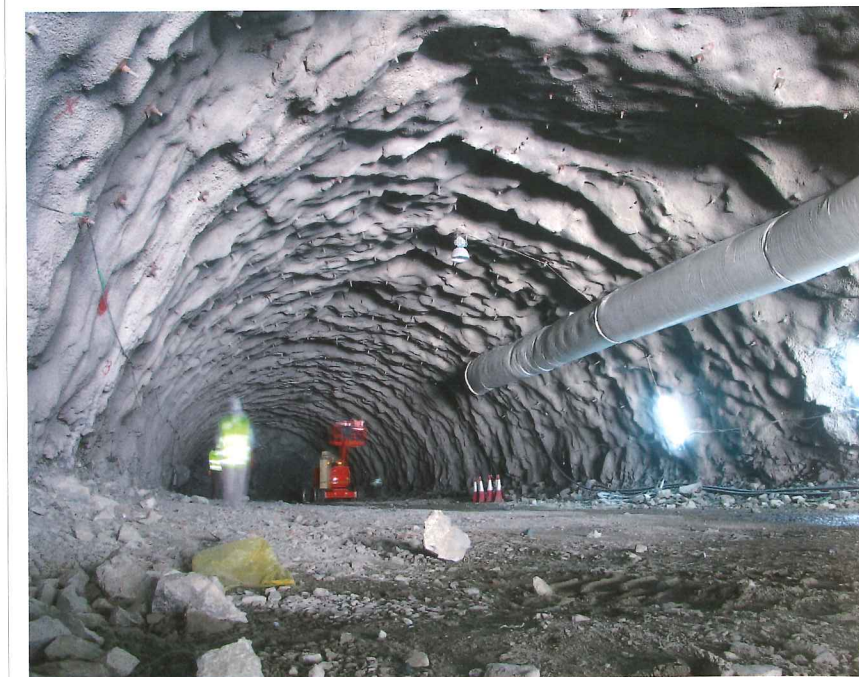
Below: NATM tunnelling for the Shis Tunnel, UAE
