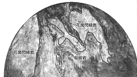
図-5 切羽状況STA.425+21.0
