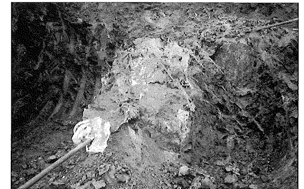
(施工例)固結状況
