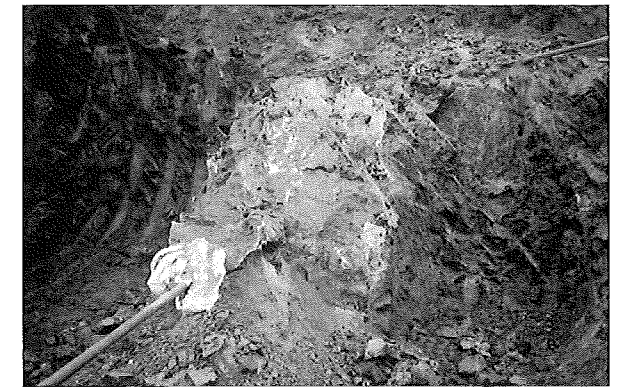
(施工例)固結状況
