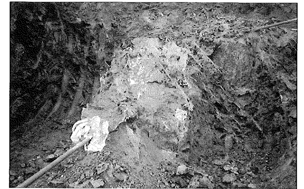
(施工例)固結状況
