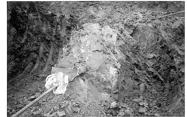
(施工例)固結状況
