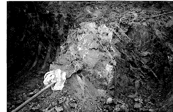
(施工例)固結状況
