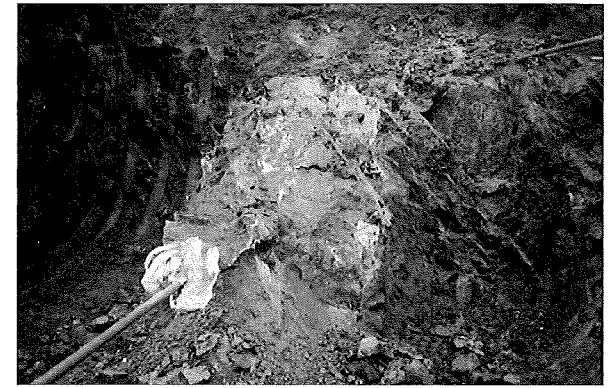
(施工例)固結状況
