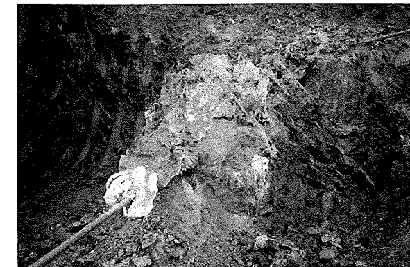
(施工例)固結状況
