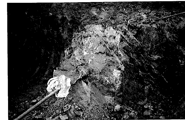
(施工例)固結状況
