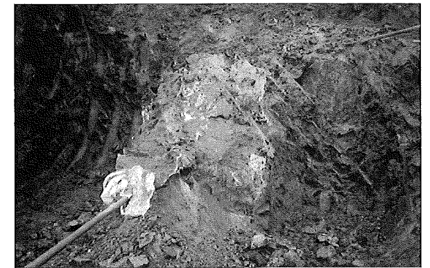
(施工例)固結状況
