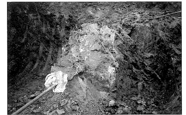
(施工例)固結状況
