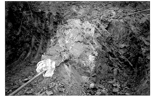
(施工例)固結状況
