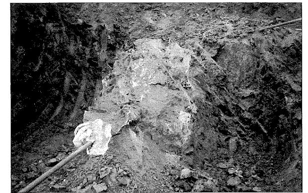
(施工例)固結状況
