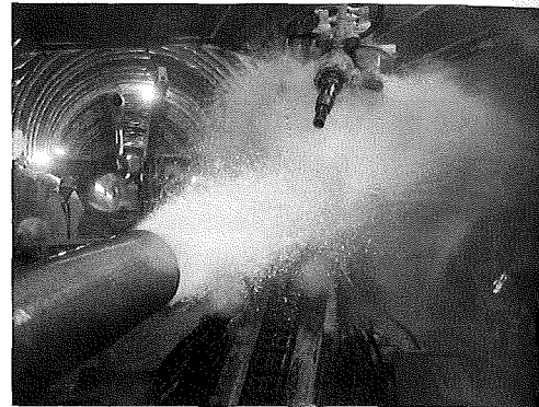
写真-11 湧水状況(2.1MPa, 5t/分)
