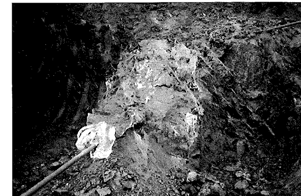
(施工例)固結状況
