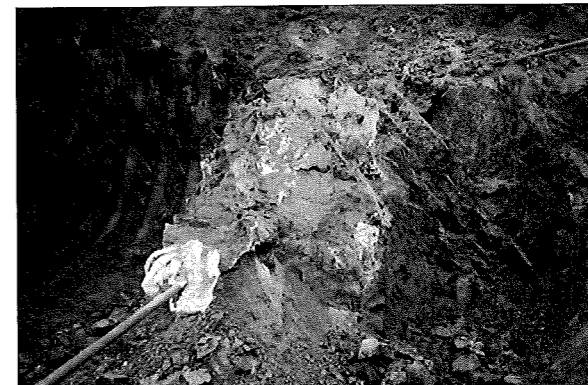
(施工例)固結状況
