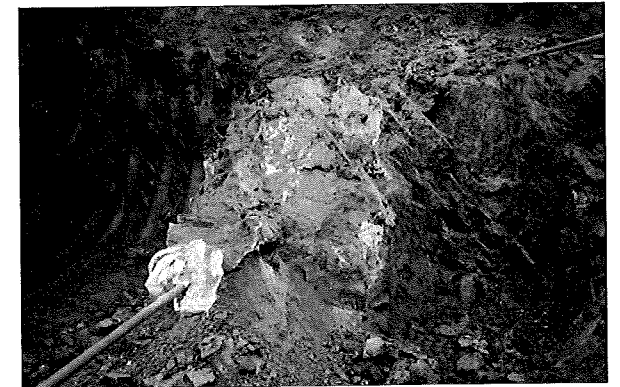
(施工例)固結状況
