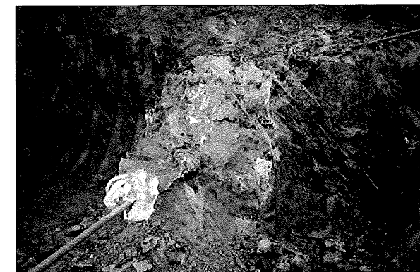
(施工例)固結状況
