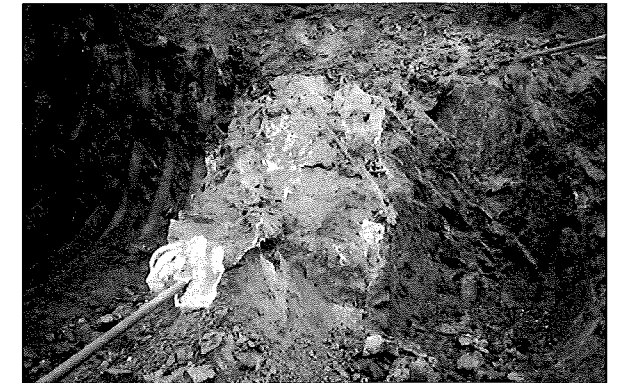
(施工例)固結状況
