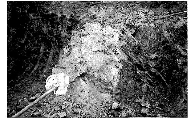
(施工例)固結状況
