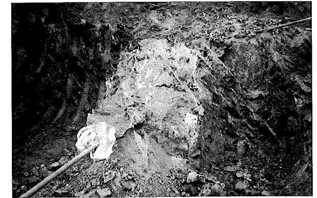
(施工例)固結状況
