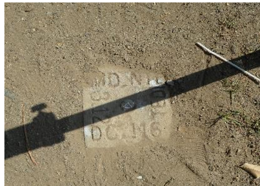
DC-116 (Hỏng nôm sứ/Damaged)
