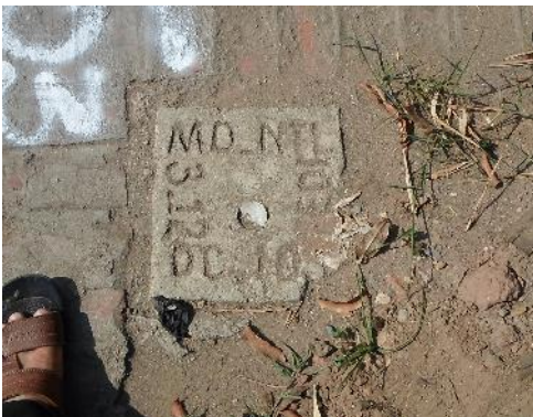
DC-103 (Hồng nôm sừ/Damaged)
