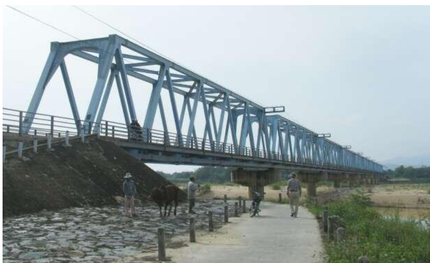
Figure 6.8 Ky Lam Railway Bridge
