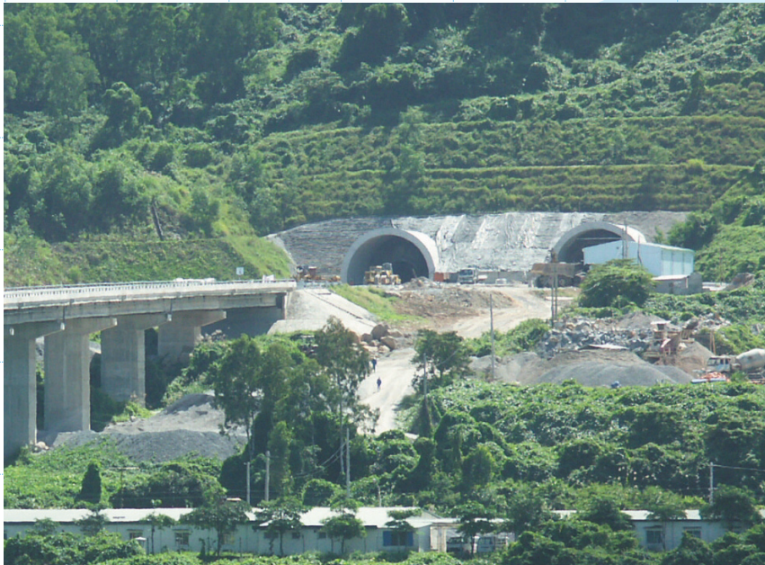
North Portal (View from North Toll Plaza)
