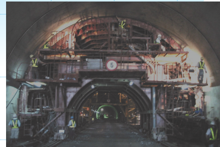
Sliding Form for the Main Tunnel (L = 12m)
