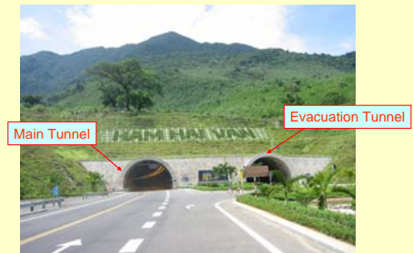
South Portal (Danang Side)
