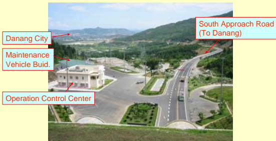
View From South Portal (Danang Side)
