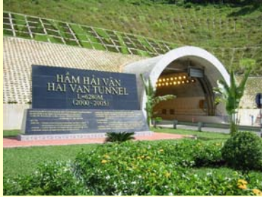
Tunnel Monument and Portal (North)
