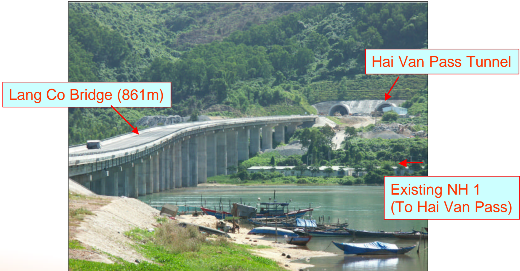
Lang Co Bridge (North Approach)
